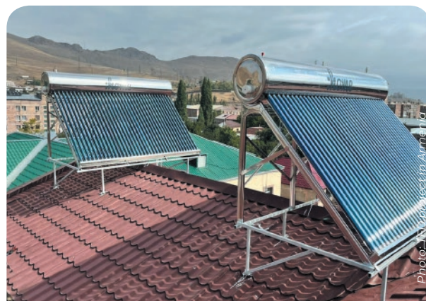
Solar water heaters at residential buildings in Armenia
